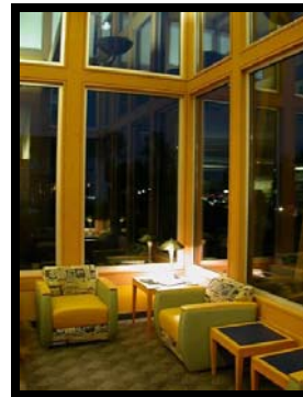
Repaired windows from the inside
